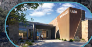
NEWLY RENOVATED EXTERIOR, LOBBY AND LANDSCAPING
