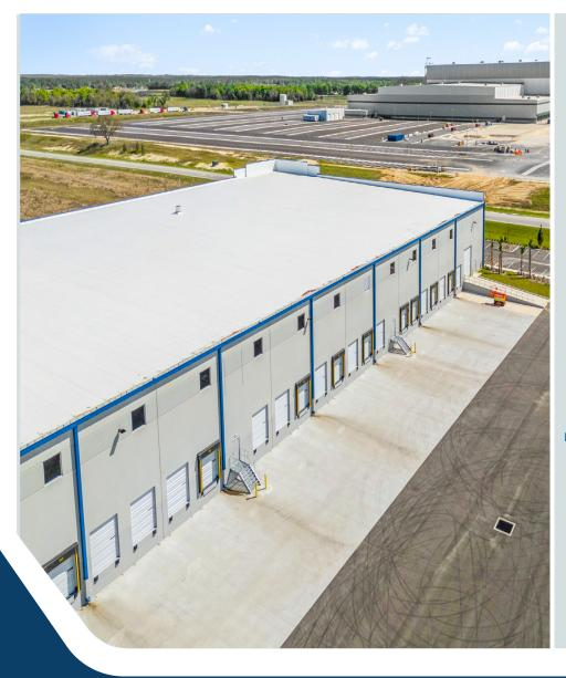
**BUILDING TYPE** Concrete Tilt Wall with bar joist & TPO roof
